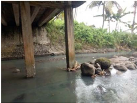
Figure 2. Damage to the Pier of the Tukad Yeh Bakung Bridge.
